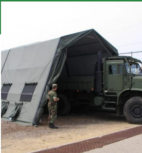
PVC operations shelters
